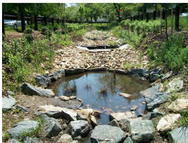
Regenerative Step-pool drainage. Photo: My Green Montgomery
