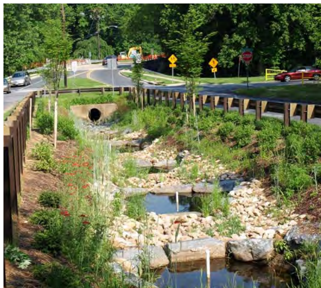
Regenerative Step-pool drainage. Photo: My Green Montgomery
